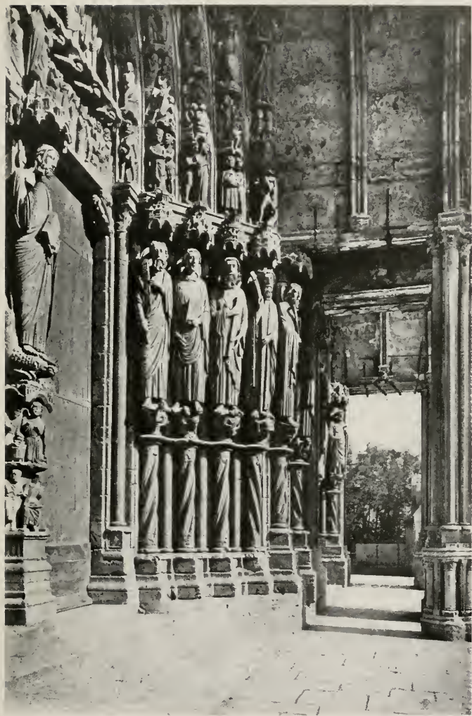
CATHEDRAL, CHARTRES, FRANCE (TRANSEPT PORCH)
